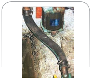
Clamps installed with screw tightening heads in line. It is recommended to offset as see below.
