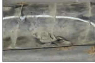
Hole in hose cover that exposes reinforcement
